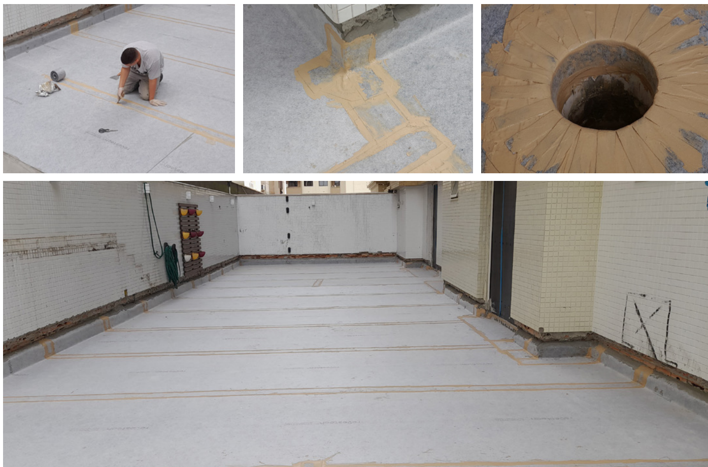
Waterproofing of 700 sqm with ECODRY120 on all exterior walkable terraces. Condominium in Itapema. Brazil.
