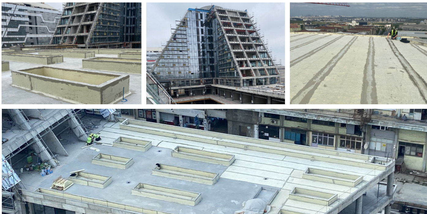
Waterproofing of 20.000 m 2 of membrane DRY120 on all walkable outdoor terraces. ISTMALL ISTANBUL. Office building, university and shopping centre. Istanbul , Türkiye.
