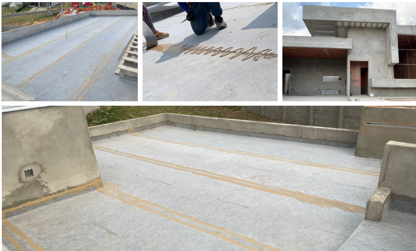
Waterproofing of 2500 sqm with ECODRY120 in luxury villas. State of São Paulo. Brazil.
