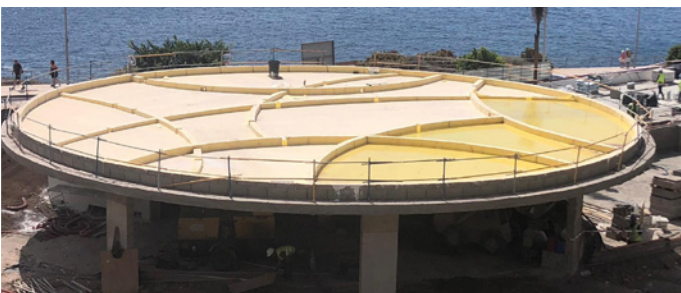
Waterproofing with DRY80 on the roof of the swimming pool bar in five star RESORT H10***** Costa Adeje. Tenerife. Canary Islands. Spain.
