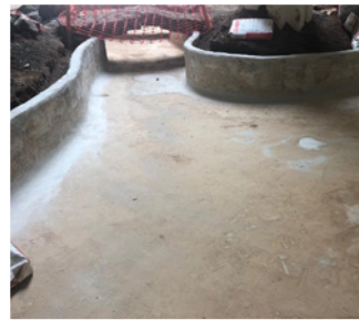
Waterproofing of terraces with DRY80 membrane. MELIÁ SALINAS***** HOTEL _ Lanzarote. Canary Islands. Spain.
