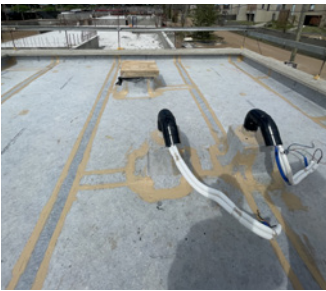
Waterproofing of walkable flat roofs with ECODRY120 . SINGLE-FAMILY RESIDENTIAL HOUSING. Montevideo. Uruguay.
