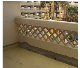
Waterproofing of terraces with DRY80 membrane. IBEROSTAR LANZAROTE PARK****. Lanzarote. Canary Islands. Spain.
