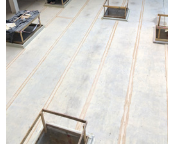
Waterproofing of 18,000 sqm with DRY120 and prefabricated tileable channel with WALK LEVEL . APOQUINDO RESIDENTIAL AND COMMERCIAL URBAN PROJECT . Santiago de Chile.
