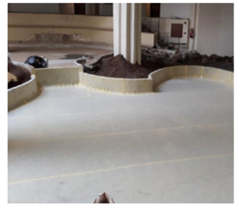
Waterproofing of terraces with DRY80 membrane. MELIÁ SALINAS***** HOTEL _ Lanzarote. Canary Islands. Spain.
