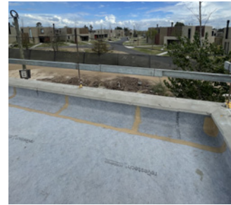
Waterproofing of walkable flat roofs with ECODRY120 . SINGLE-FAMILY RESIDENTIAL HOUSING. Montevideo. Uruguay.
