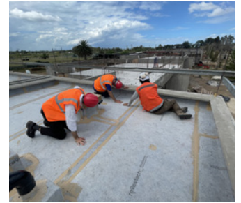
Waterproofing of walkable flat roofs with ECODRY120 . SINGLE-FAMILY RESIDENTIAL HOUSING. Montevideo. Uruguay.
