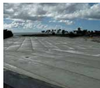
Waterproofing of 8.000 m 2 of flat wakable roofs with DRY80 . Hotel SAINT REGIS Cap Cana. Dominican Republic.
