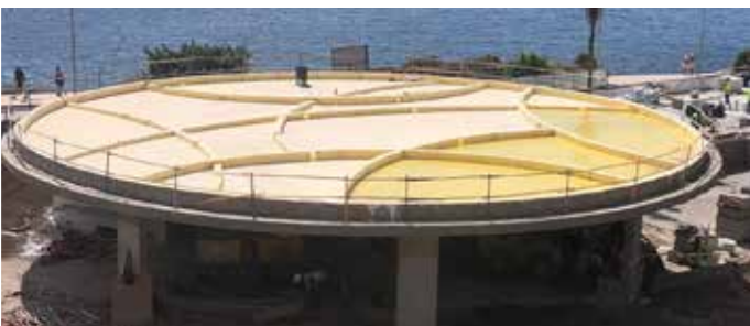
Waterproofing with DRY80 of the pool bar roof of the 5-star resort CHAIN H10_Costa Adeje, Spain.
