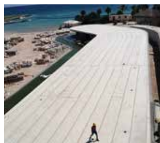
Waterproofing of 8.000 m 2 of flat wakable roofs with DRY80 . Hotel SAINT REGIS Cap Cana. Dominican Republic.
