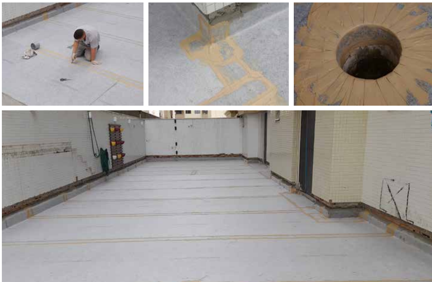
Waterproofing of 700 m 2 with ECODRY120 on all its outdoor walkable terraces. Condo in Itapema. Brazil.
