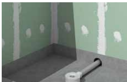
CONNECTION OF THE DRAIN
