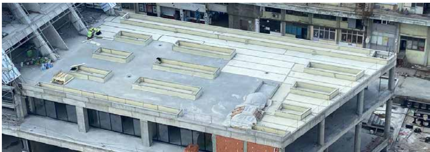
Waterproofing of 20.000 m 2 of DRY40 and DRY120 in all its outdoor walkable terraces. ISTMALL ISTANBUL. Building for offices, university and shopping center. Istanbul. Turkey.
