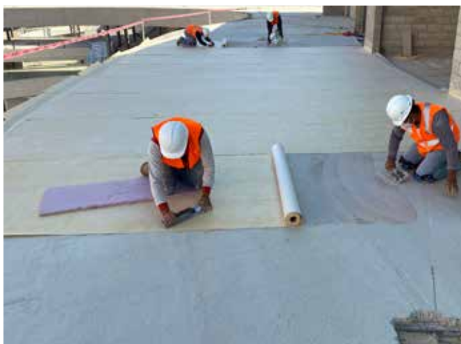
Waterproofing of 35.000 m 2 of DRY120 in all its outdoor walkable terraces. PLAZA PENINSULA MALL. Tijuana. Mexico.
