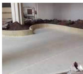
Waterproofing of the interior gardens with DRY80 designed by César Manrique. Hotel MELIÀ SALINAS Costa Teguise. Tenerife, Spain.
