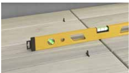
INSTALLATION OF THE BATHROOM FLOOR
